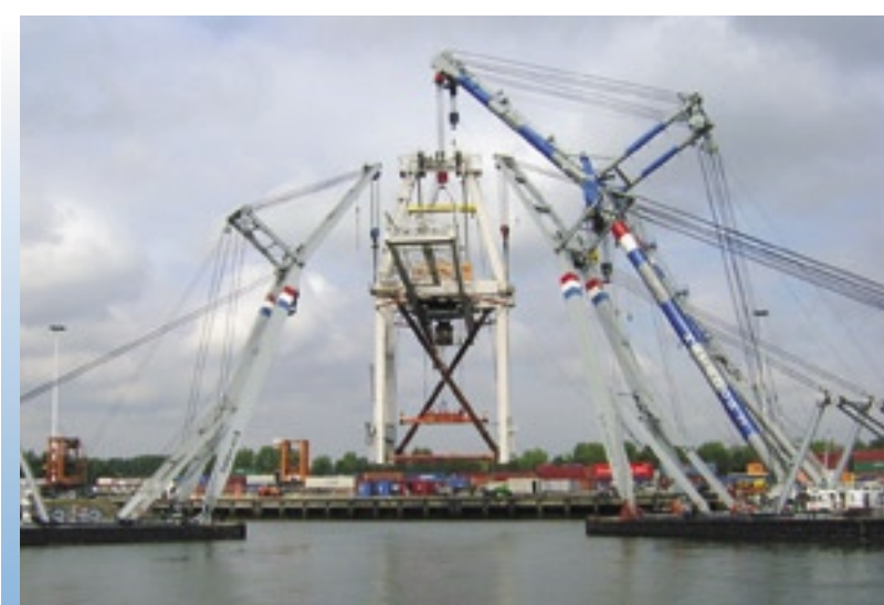
The three sheerlegs move the crane over the water and split up their positions so the pontoon can be positioned underneath the crane.
