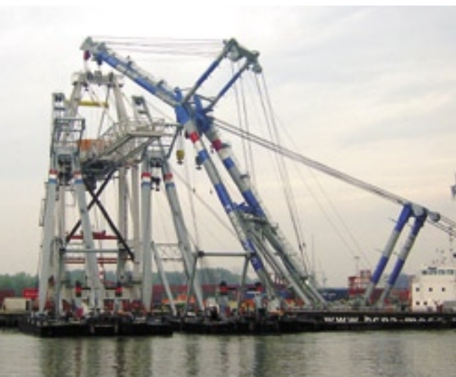
Three sheerlegs connecting to the crane on the quay.
