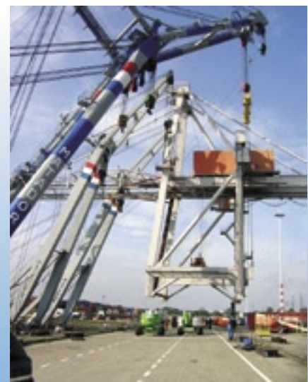
Here, the original extension pieces are removed from the crane.
