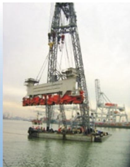
Bringing the bogies to the pontoon with sheerleg number 4.
