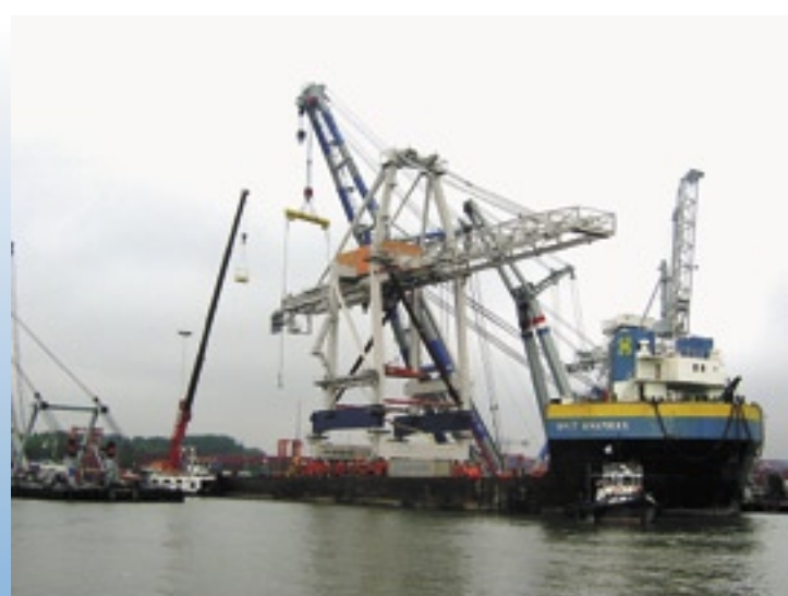
The result: a crane of the same height, but with a railspan of 20m instead of 15m.
